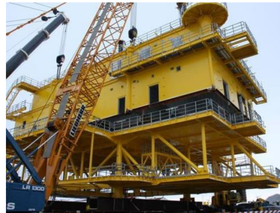
Steel structures fabrication
