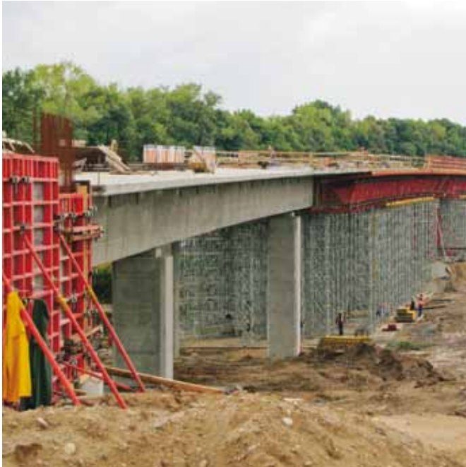
Construction of a western ring road in Mrągowo.
