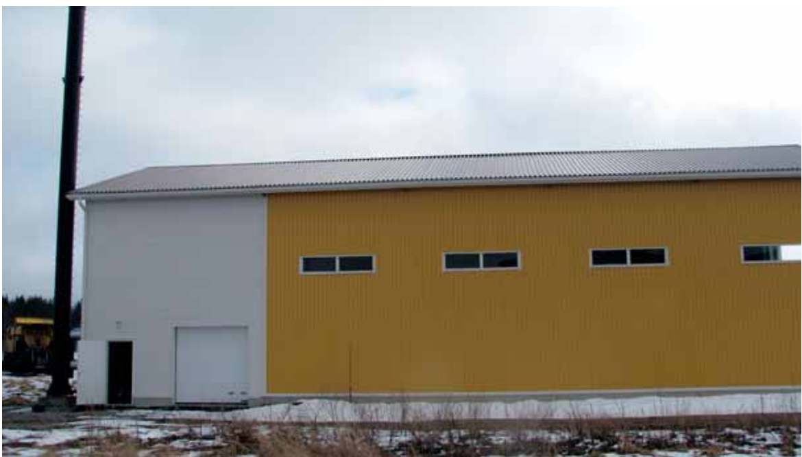
Agricultural biogas plant
